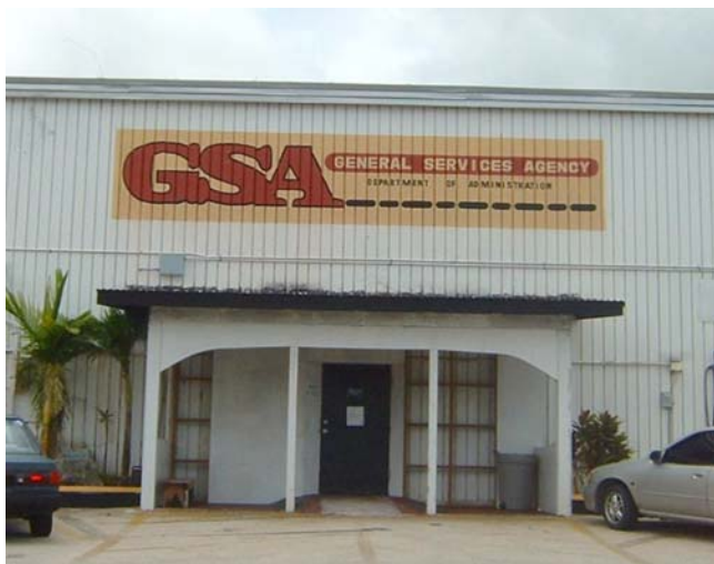
External view of General Services Agency.
