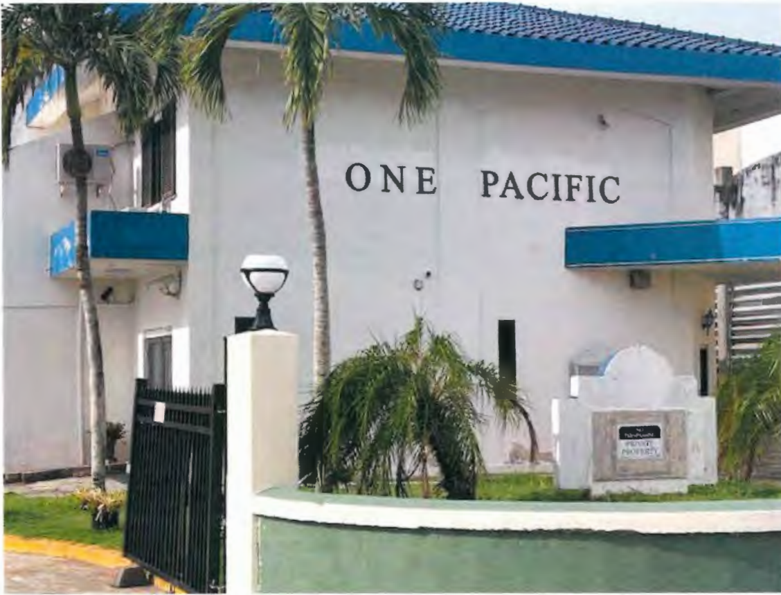
Condo complex on East Boundary
