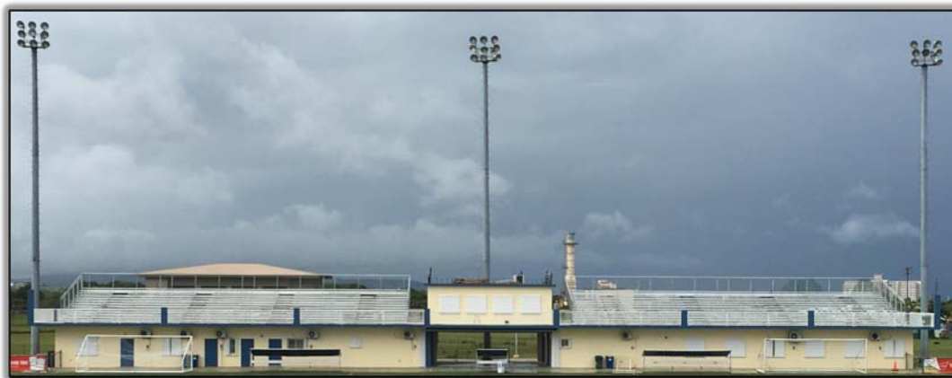
Image 6: Northern Soccer Stadium – Newly constructed GFA National Academy Center.
