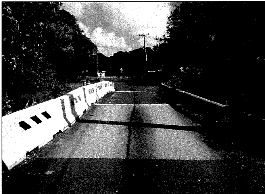
Photo no. 2 Deck overview looking west
