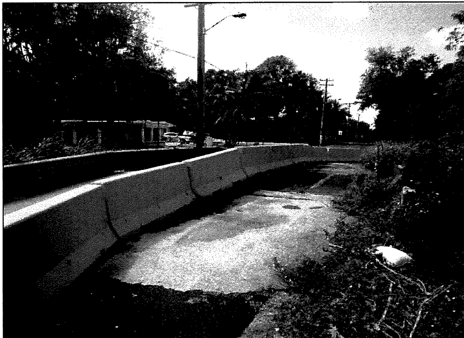
Photo no. 4 Non-traffic side of bridge on downstream end
