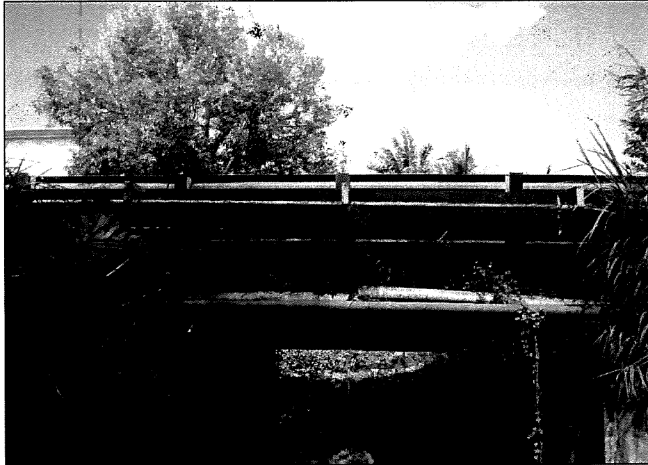
Photo no. 3 Elevation view from upstream
