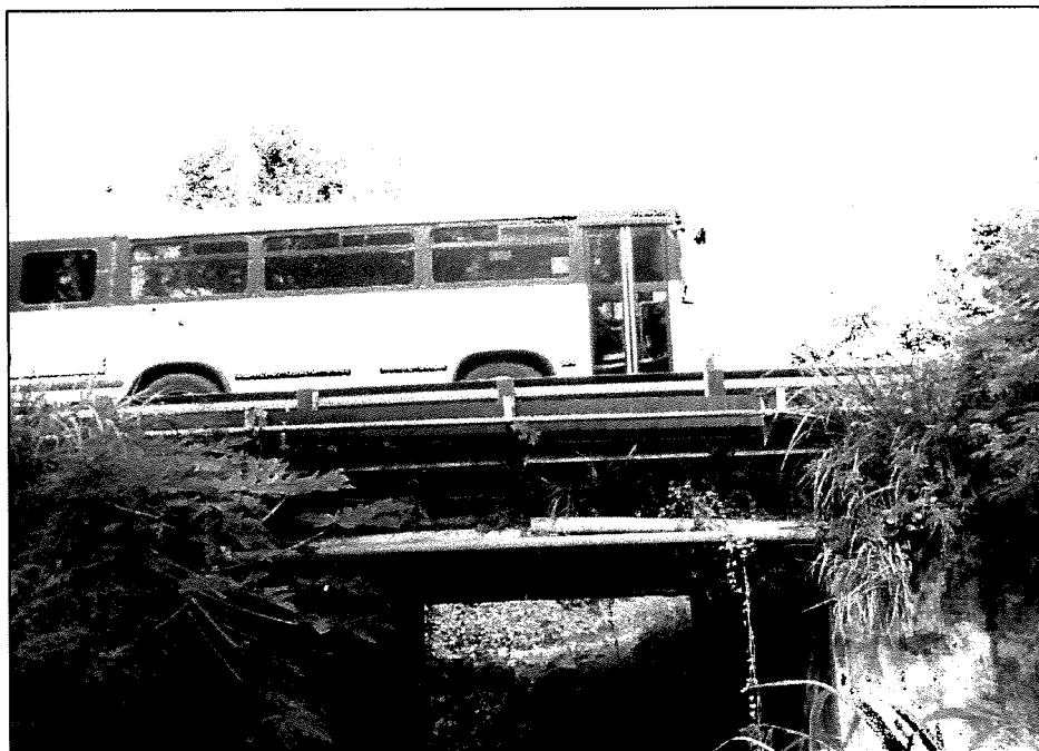
Photo no. 11 Passage on Pigua bridge by MRT bus
