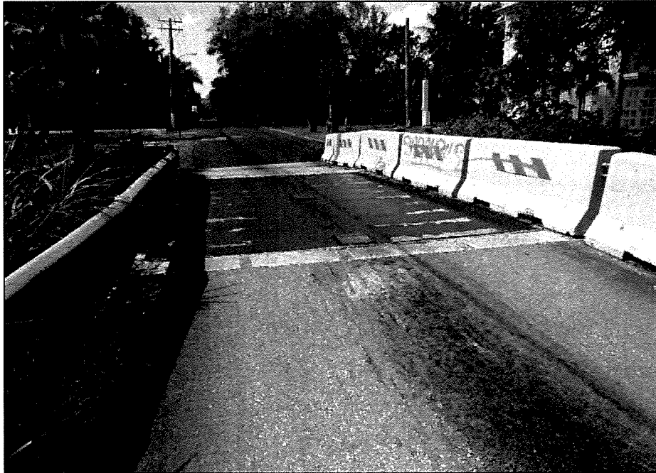
Photo no. 1 Deck overview looking east
