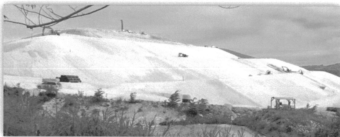
Figure 7 West side soil protection layer complete (March 2015)
