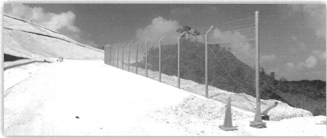
Figure 12 Perimeter Security Fence
