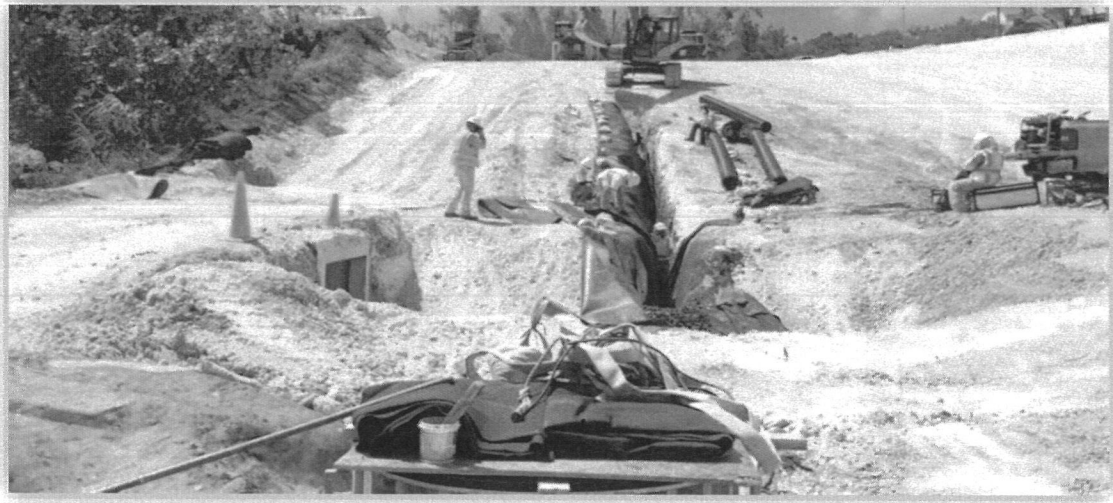
Figure 10 West side leachate perimeter collection trench installation
