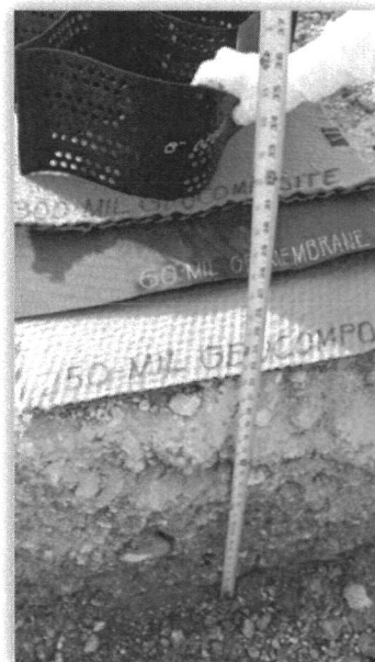
Figure 3 Landfill cover layers as they are constructed
