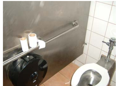
Photo 5: Inside one of the restrooms at the Chamorro Village.
