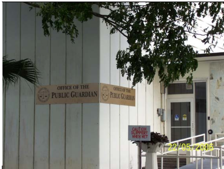
Image 1: Office of the Public Guardian Building in Hagatna
