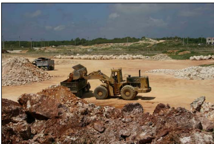
Image 1: Earth-moving equipment at the Guam Raceway Park
