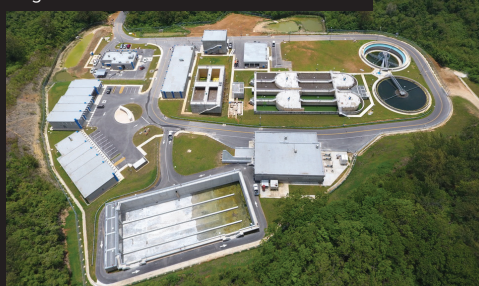
Agat-Santa Rita Wastewater Treatment Plant
