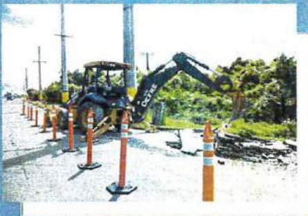
DPW road paving project at Mongmong
