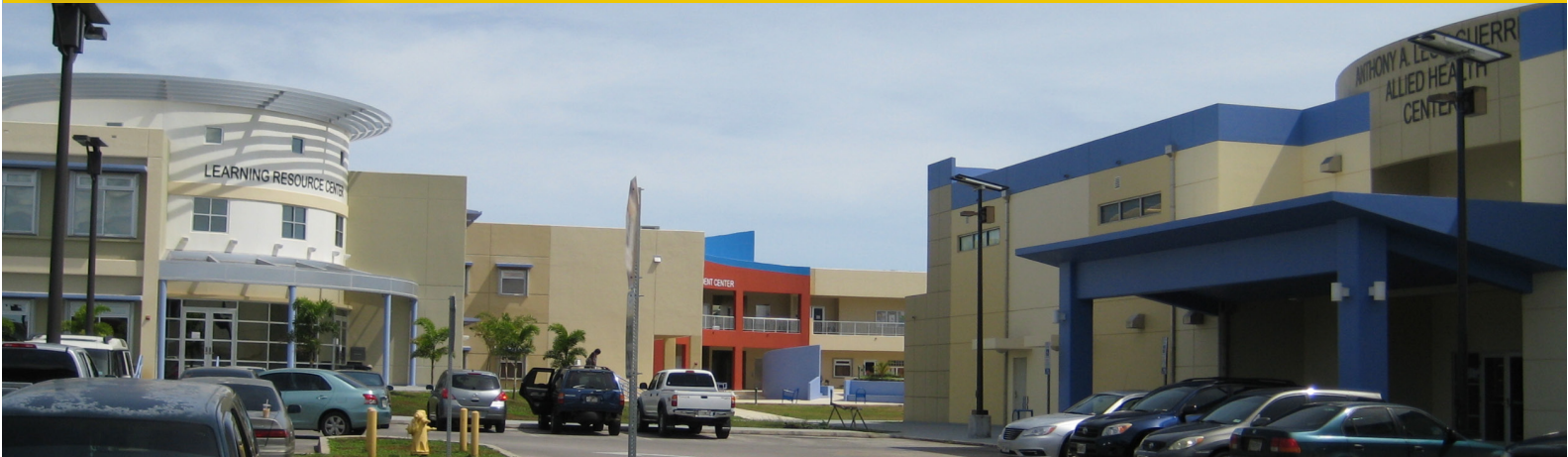
GCC has added three new buildings to its campus over the past three years: the Anthony A. Leon Guerrero Allied Health Center (right) in 2009, the LEED-Gold certified Learning Resource Center (left) in 2010, and its new Student Center (center) in 2011.
